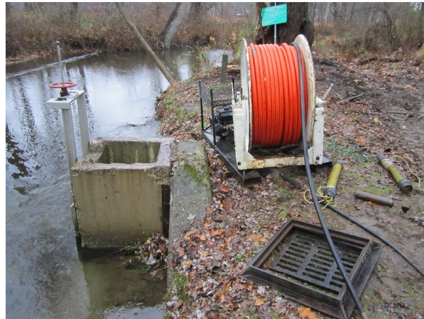
EXISTING OUTLET STRUCTURE
